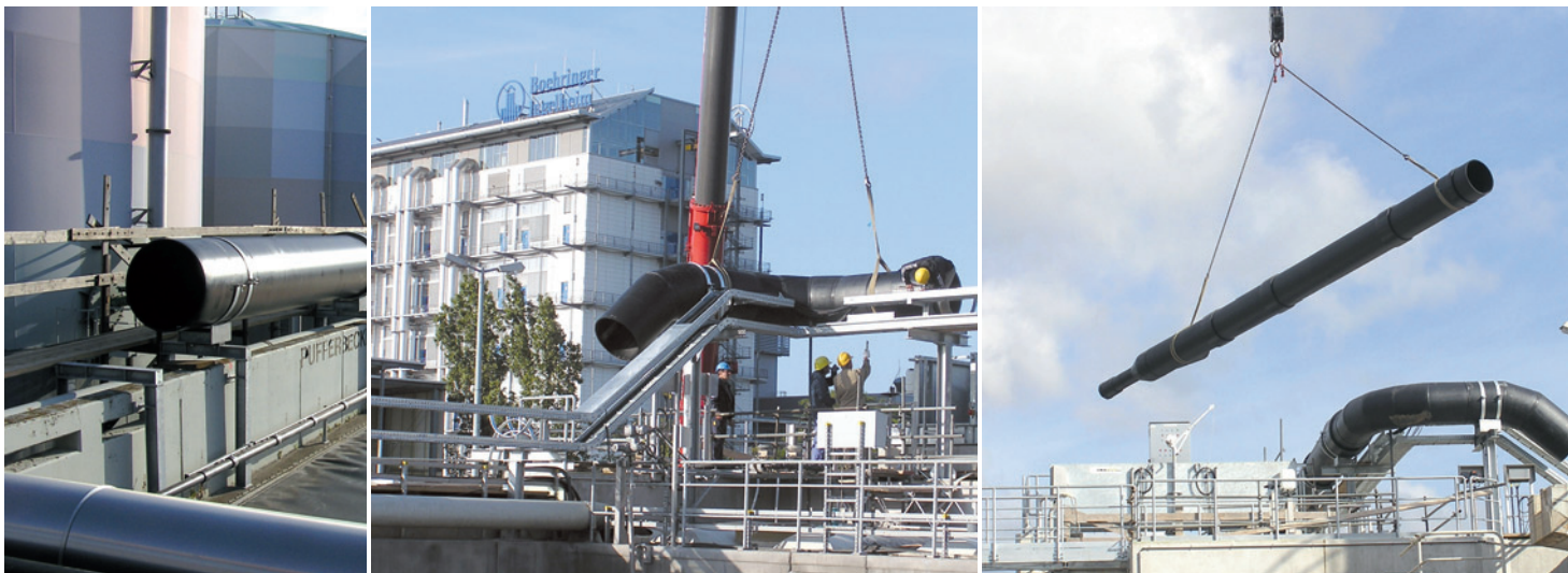
The pipes are secure on a network of pipe bridges. Numerous custom components make it possible to meet the particular conditions.
