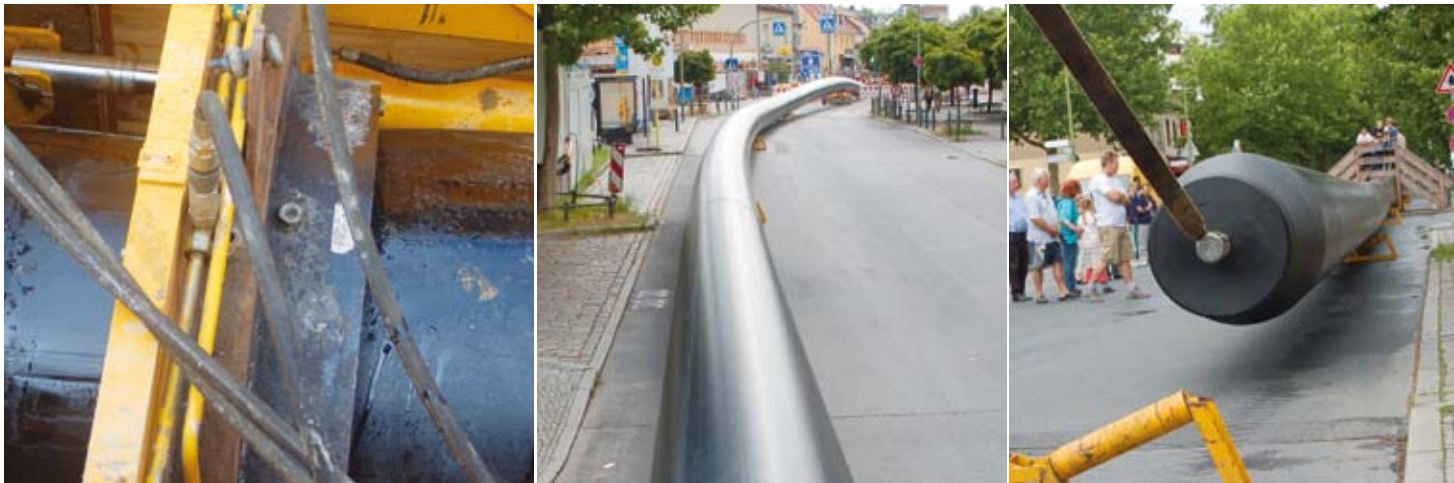
Left: The reducing tool brought down the circumference of the SIMONA® PE 100 pipe from 1060 mm to approx. 970 mm. Middle: The 500 m long pipeline was drawn into the old pipe in a single feed. Right: The entire pipeline was transported to the access trench with light.
