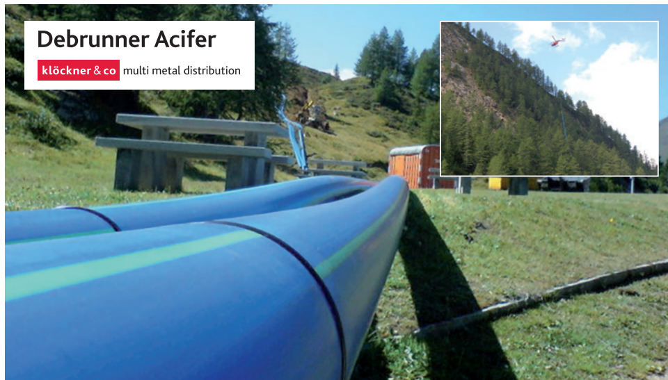
Rough terrain calls for pipes with properties that provide maximum protection. Pipe trains measuring 60 metres in length were transported by helicopter.
