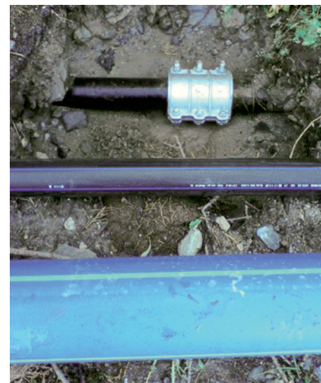
The 40-year-old cast-iron pipe (top) is replaced by a new pressure pipe (bottom); a provisional pipe made of PE (centre) ensures temporary supply.
