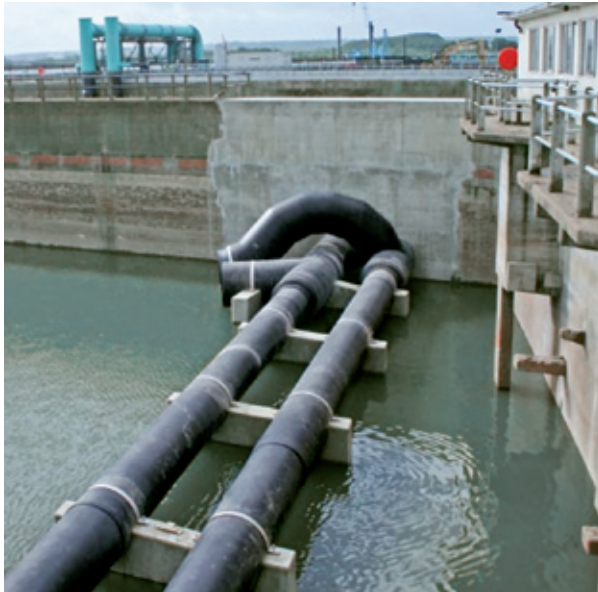
l: Feed lines made with large-size SIMONA® PE 100 pipes; t. r. Brackish water storage tank with PE 100 feed pipe, OD 1000/1200 mm; d. r. Raised PE 100 collecting main below the filtration modules
