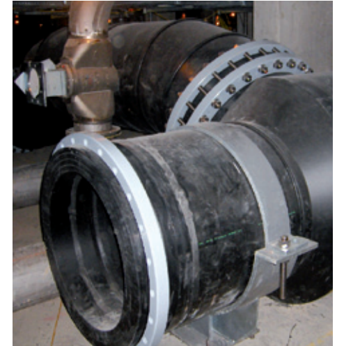
PE 100 welded pipe section, OD 900 mm SDR 17 incl. reinforced tee PN 10.
