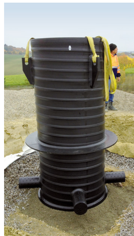
SIMONA landfill gas filter during installation
