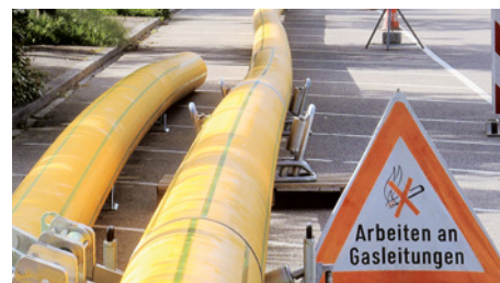
Pre-welded train of pipes ready for pipe insertion
