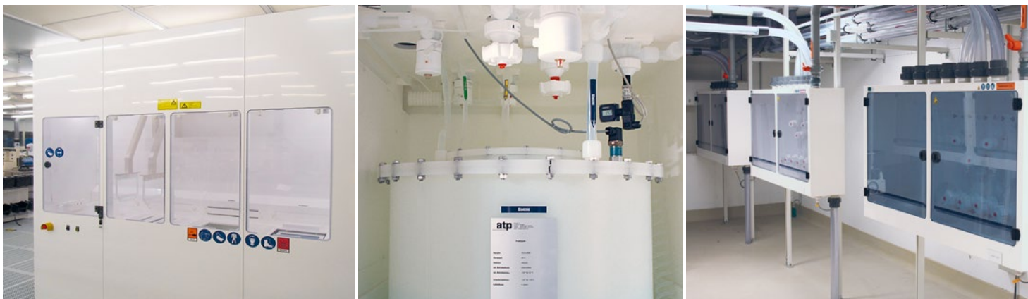
From left to right: automated wet-processing unit; interior view of the chemical supply system; distribution systems for equipment ports
