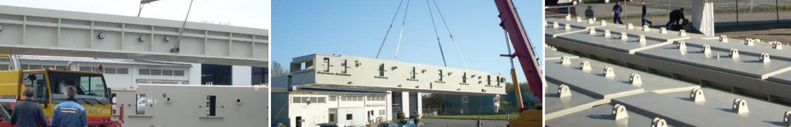
Delivery of the pickling tanks to the Rasselstein steel plant
