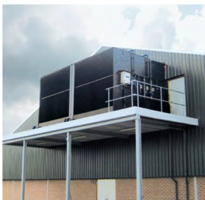
Air scrubber made of SIMONA® PE 100 twin-wall sheets, pipes and fittings
