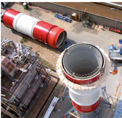
Chimney lining made of SIMONA® ECTFE-GK sheets
