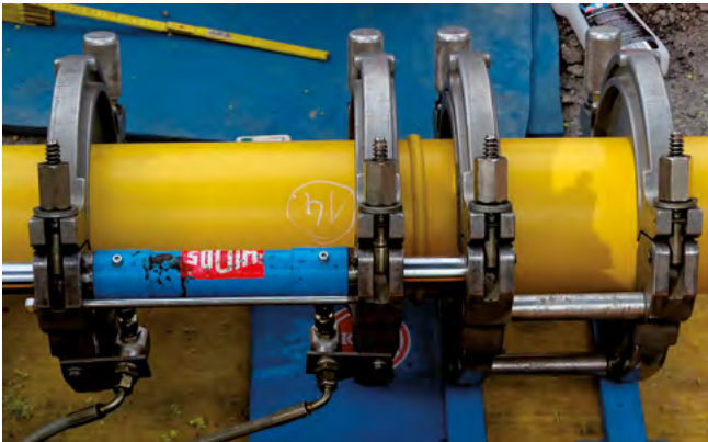
Welding a SIMONA® PA 12 gas pipeline
