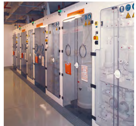
Chemical supply systems with doors made of SIMONA® PVC-GLAS
