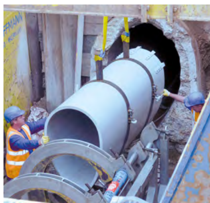
Rehabilitation of a sewer using SIMONA® PE 100 light grey ovoid pipes
