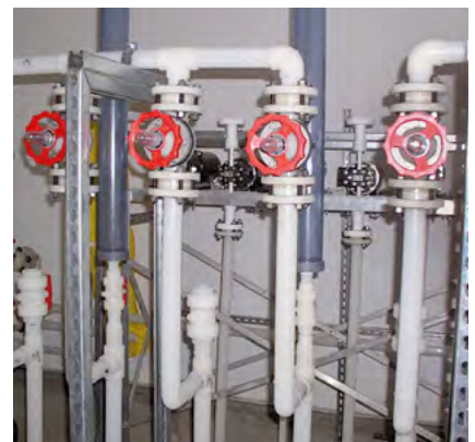
SIMONA® PVDF pipes and fittings in a water fluoridation system
