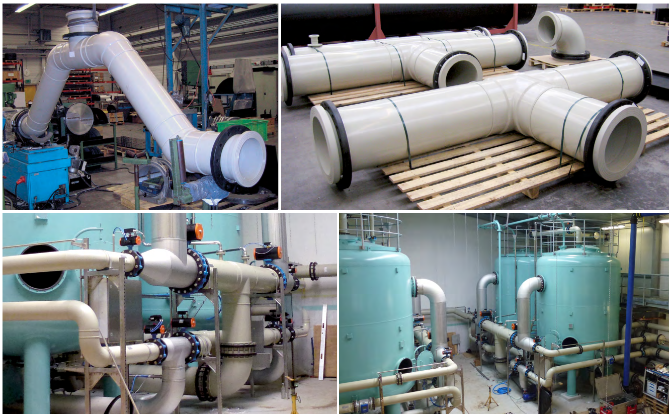
Piping system made of SIMONA® PP-H AlphaPlus® for a well water treatment plant (aerator, iron and manganese removal filters) for drinking water supply
