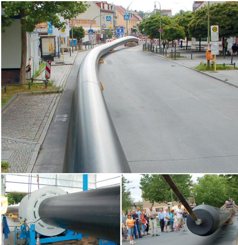
Top: The 500 m long pipeline was drawn into the old pipe in a single feed.
