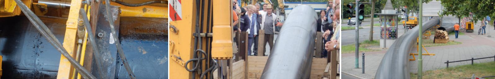
Fig. from left to right: The reducing tool brought down the circumference of the SIMONA® PE 100 pipe from 1060 mm to approx. 970 mm. Small access and exit trenches guarantee minimal disturbance for residents and traffic. The high flexibility of the SIMONA® PE 100 pipes also enabled narrow curve radii.
