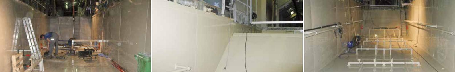
From left to right: applying the SIMONA® PP AlphaPlus® lining to the cathodic electrocoating bath; bath overflow; installing the nozzle pipes
