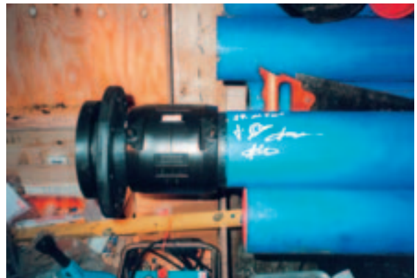
Preparation of flange connections by means of electrofusion welding
