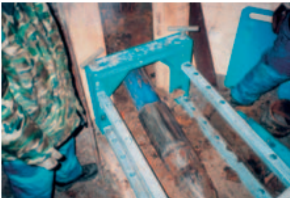
Arrival of the pipe in the reception shaft
