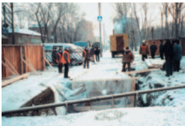
Prepared launch and working shaft
