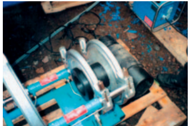
Preparation of fittings for the house connections by means of heating element butt welding
