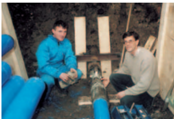
Pulling the protective jacket pipe into the old steel pipe
