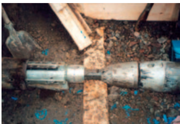
Bursting head with cutting and displacement unit being placed in the old steel pipe
