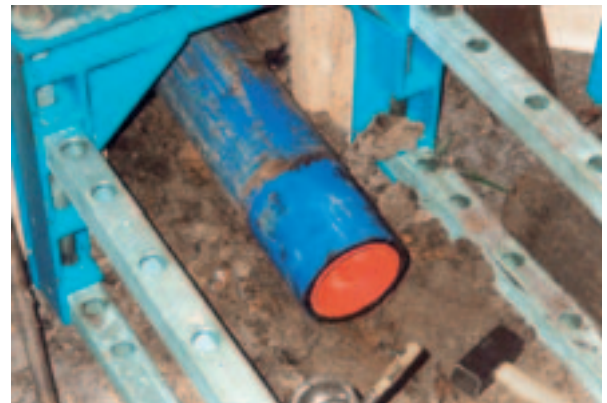
SIMONA® SPC protective jacket pipe in the reception shaft
