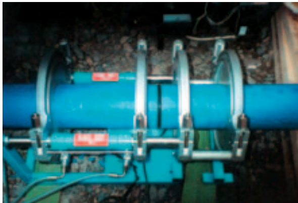
Welding d 160 x 14.6 mm, SDR 11 pipes by means of heating element butt welding. The protective jacket is removed from the welding zone with the help of a SIMONA stripping tool
