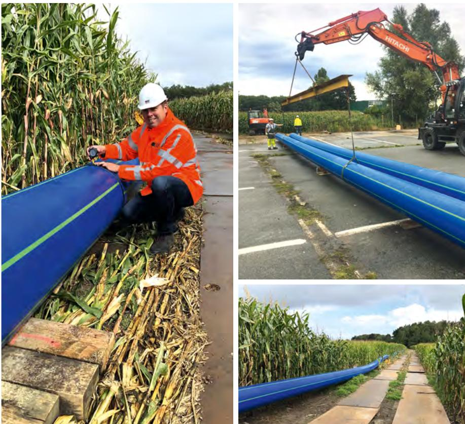
Left: Before pipe insertion, the pipes are accurately measured and checked. Top right: Transporting the 20 m long pressure pipes to the site. Bottom right: The total length renovated by horizontal directional drilling was about 740 m.
