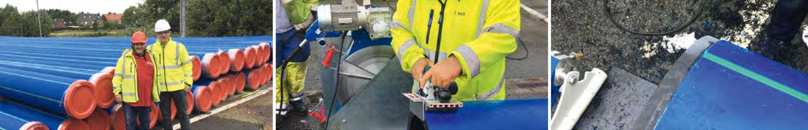
From left to right: SIMONA® PE 100 SPC RC-Line protective-jacket pipes; jacket cut-back for preparation of butt welding; pipe with jacket cut-back prepared for the welding process.
